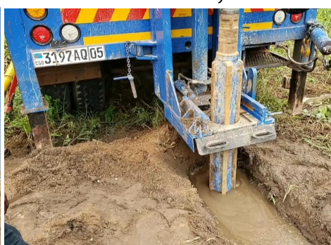
Well drilling auger beginning to turn
