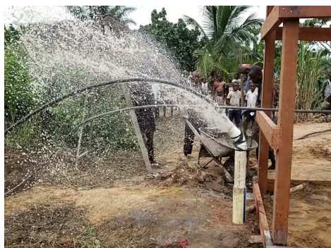
Blowing out the well for impurities
